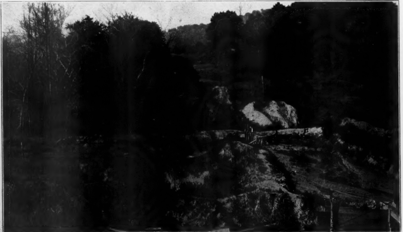
Bird's Eye View of Two of the Settling Tanks. Cedar Grove
